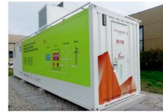
Figure 2.1: The 720kVA/500 kWh grid-connected BESS installed at the EPFL campus
