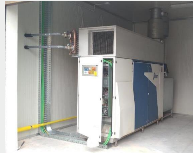
Microturbine T100 and inlet heat exchanger
