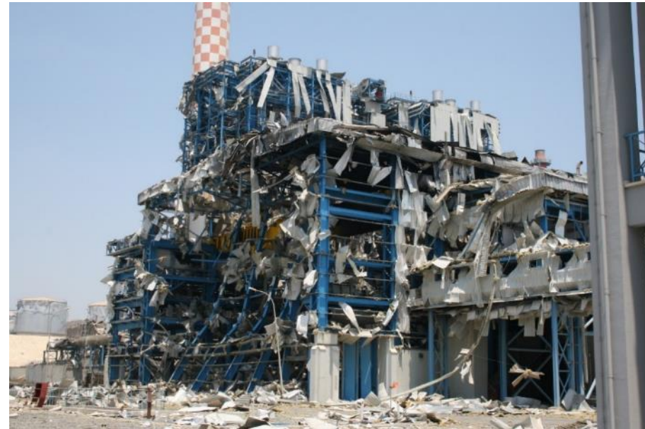
Vassiliko Power Station, 2 days after the explosion in July 2011
