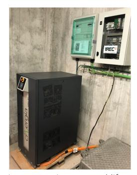
**Demo site:** Montgat library with photovoltaics generation, second life battery and smart heating, ventilation, and air conditioning management system
